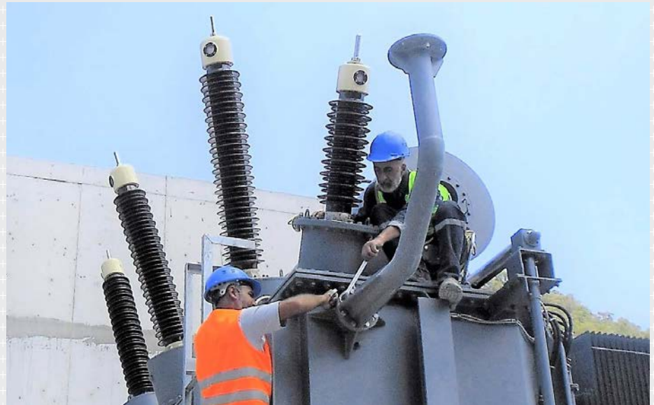
170 kV & 72.5 kV YASH OIP bushings. Transformer: Hyundai Heavy Industries. Site: Geothermal Power Plant – Turkey.
