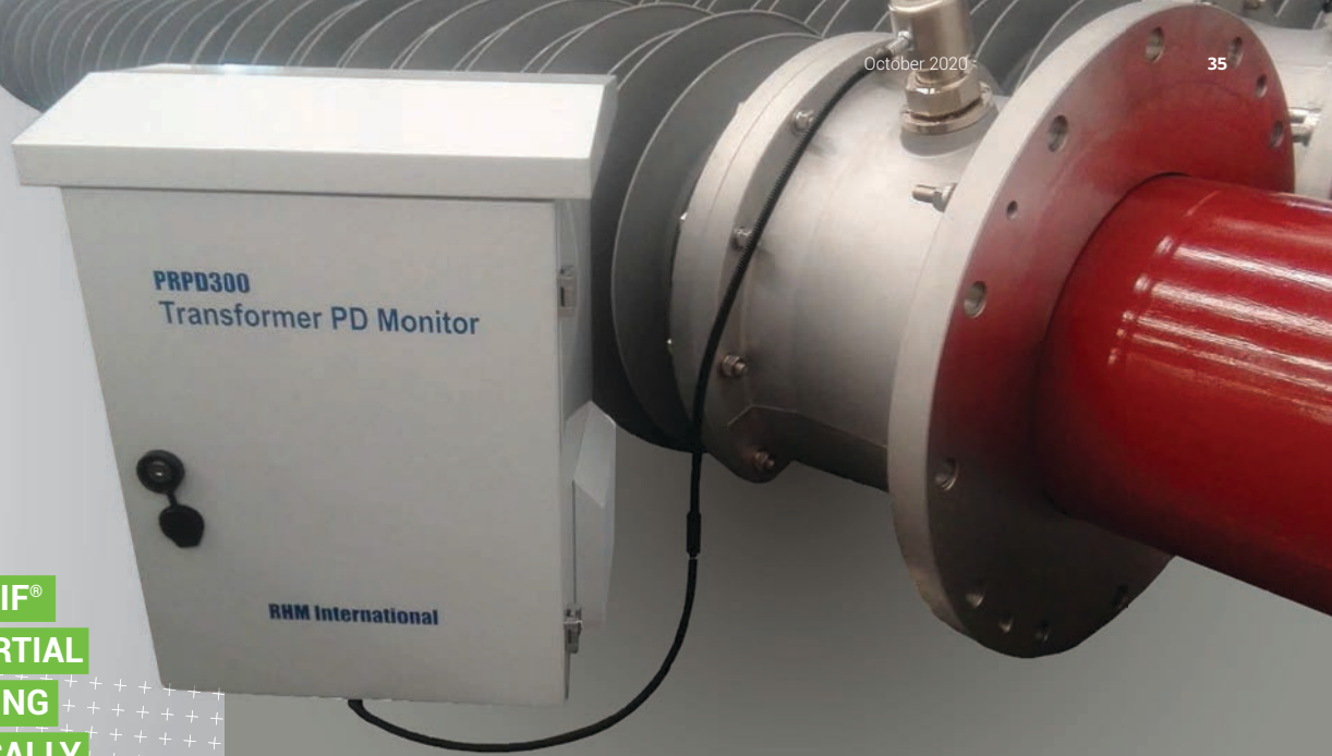
Figure 3. RIF® bushing with smart terminal and PD sensor
